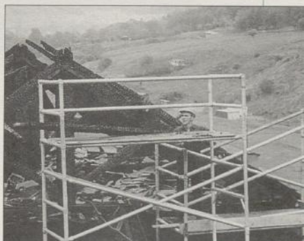
Re-roofing Cwmparc Workingmen's Hall after a fire in 1987.
